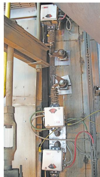
LP20 Pneumatic Linear Actuators with AV Positioners Installed on Windbox Dampers
